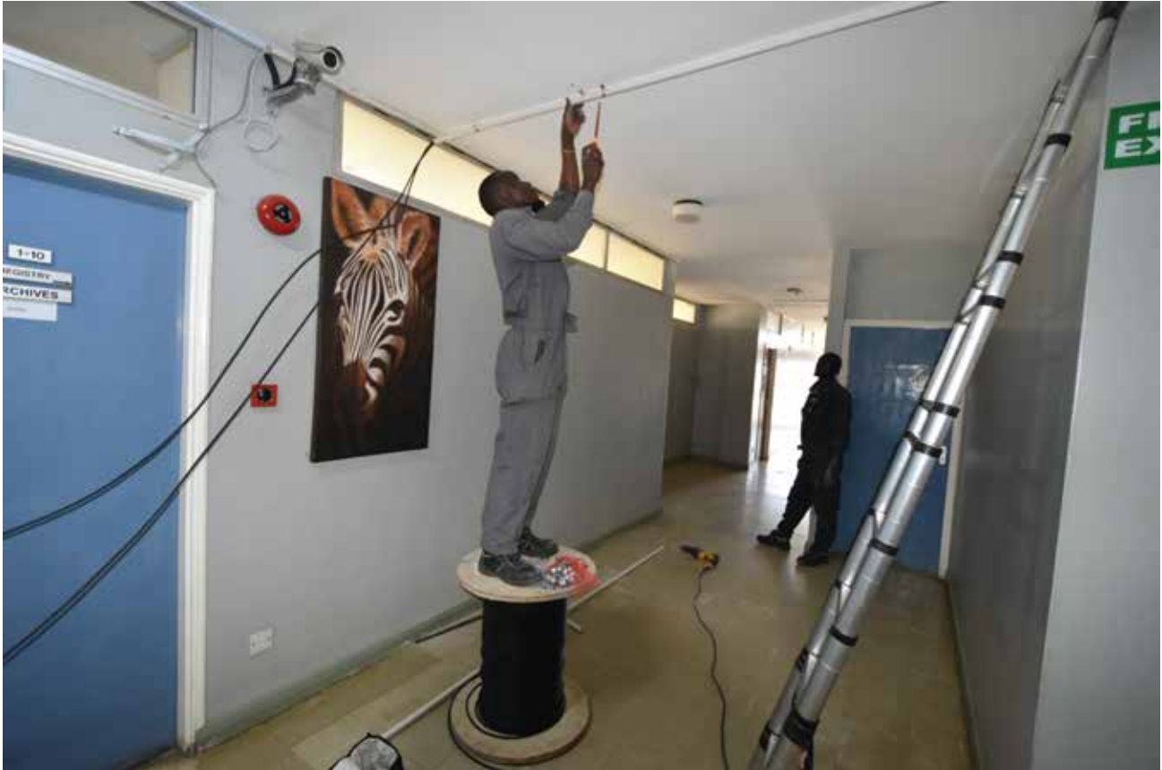
Technicians setting up cables at KLB Head Office.
