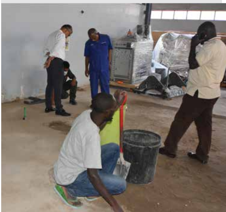
The ongoing floor preparations
